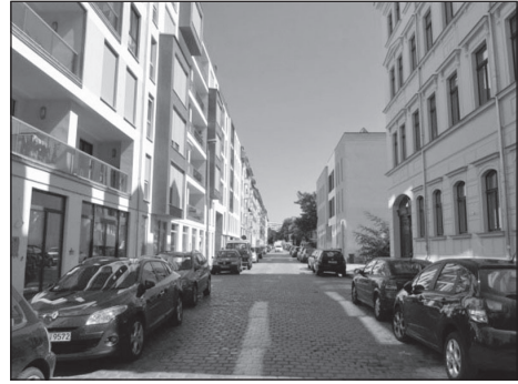
Fig. 9 – New multistory construction. Photo: D. Rink.
