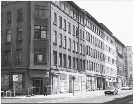
Fig. 4 – Dilapidating inner-city housing stock. Photo: A. Haase.
