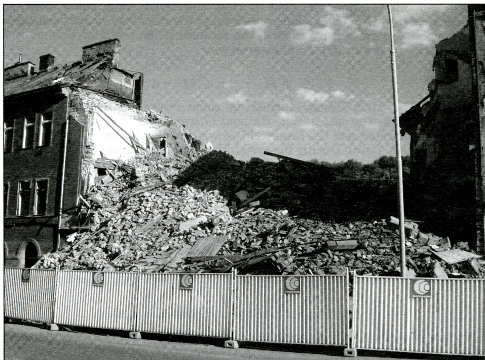
Fig. 2 – Collapsed building in Karlín (summer 2002)
